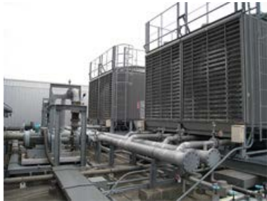
Cooling Water Pump equipment
