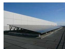
Solar generation equipment in Kawagoe plant
