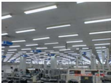
Replacement to straight LED lamps
