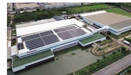
An array of solar panels on our plant's rooftop in Thailand
