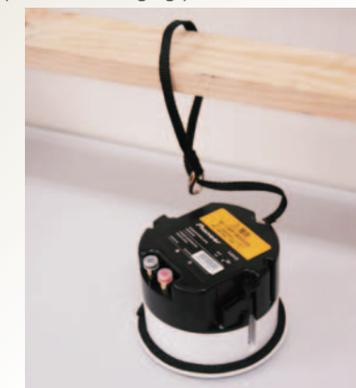
Example: A ceiling mount speaker fitted with an additional safety wire as a precaution against a fall
