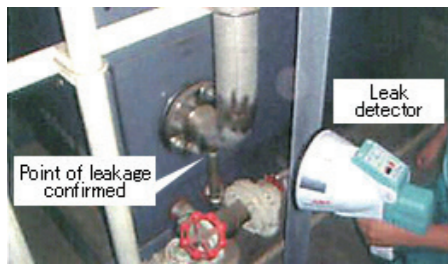
Air leak inspection
