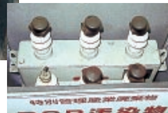
High-voltage condensers in storage
