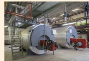
Two large boilers (example)
