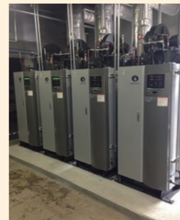
Four high-performance compact boilers
