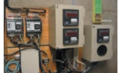
A Power Consumption Measurement System Installed at the Headquarters
