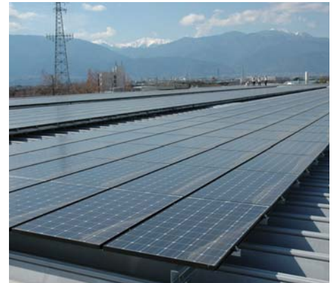
Hybrid photovoltaic generation panels
