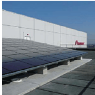
Photovoltaic system at Pioneer's Kawagoe Plant
