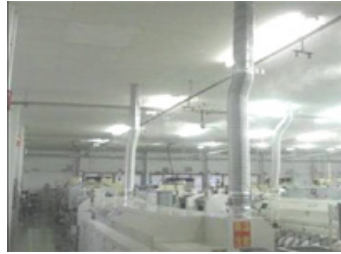
Reflow furnace area
